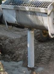
**STEP1: LOADING** of the inert material is made directly with the mixing bucket attached to the machine. In the second stage water & cement is added in the proportions necessary
